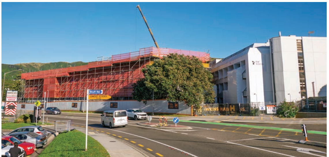
Construction of the Kenepuru Science Centre for PHF Science, Wellington.
