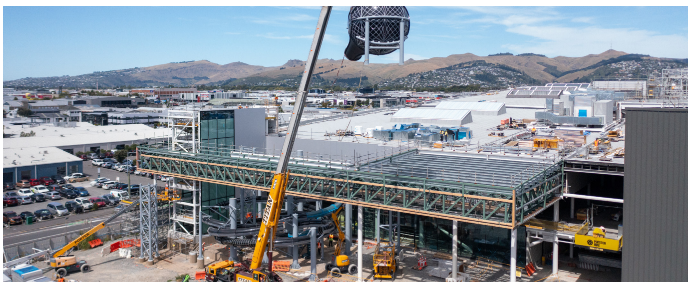
Hydroslide installation at Parakiore
